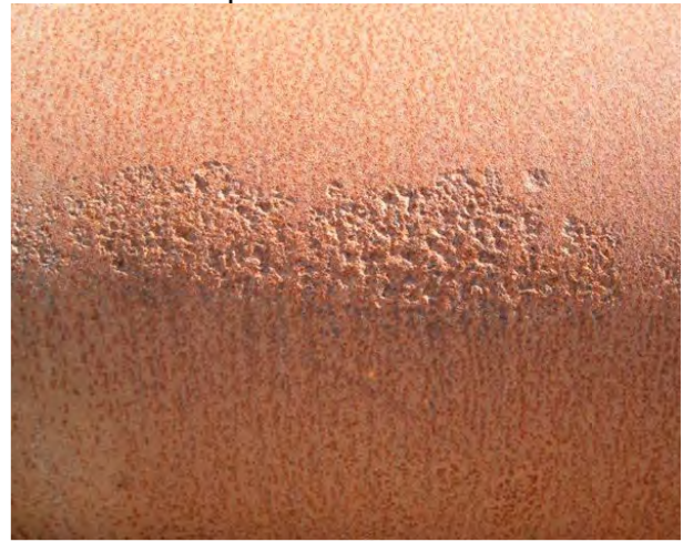
d) Fasciame serbatoio GPL
